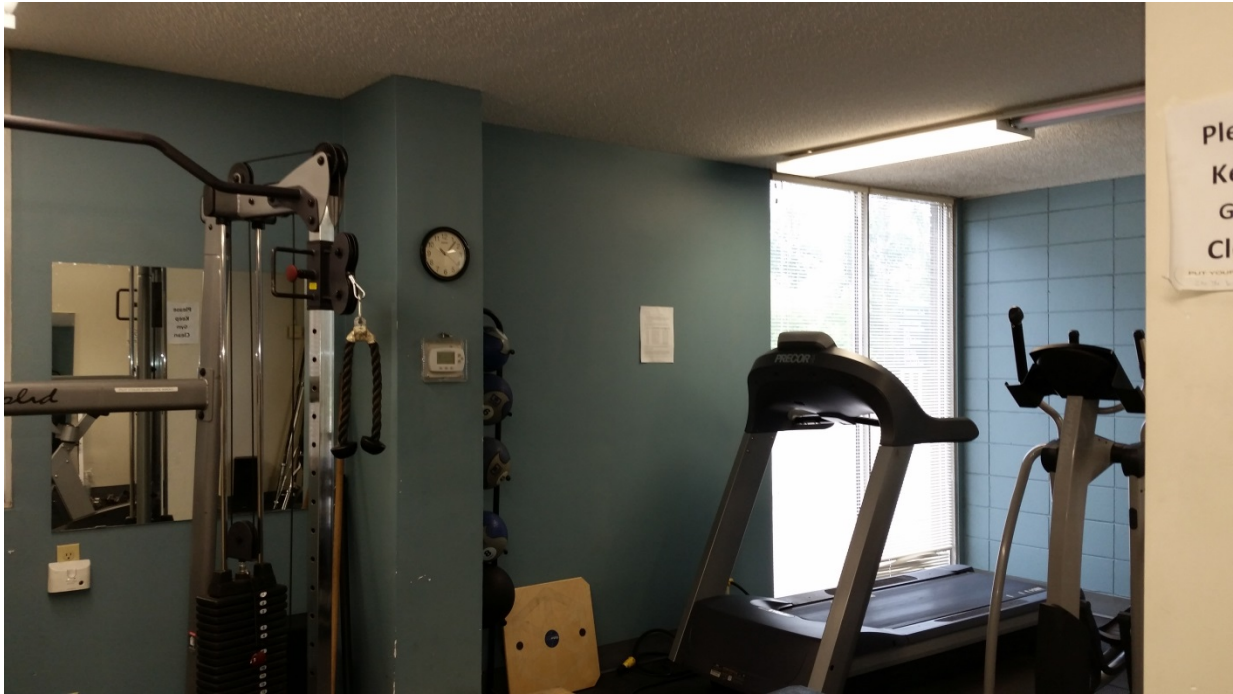
Photo 17 – Fitness Room Lighting
