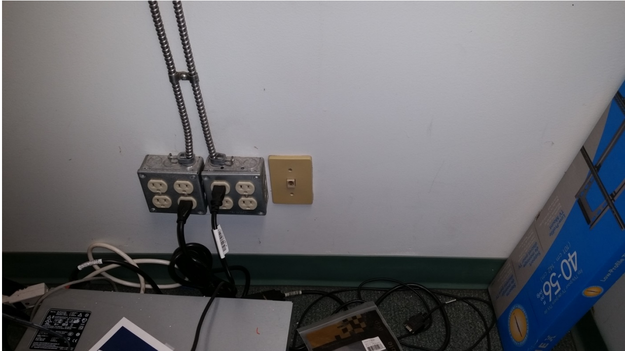
Photo 20 – New Surface Mounted Receptacles Fed From BX
