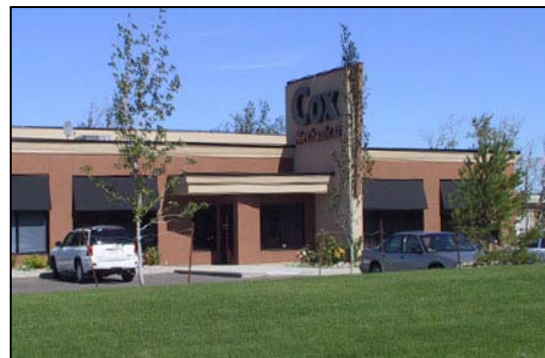
A parapet on the roof effectively screens roof-mounted equipment.
