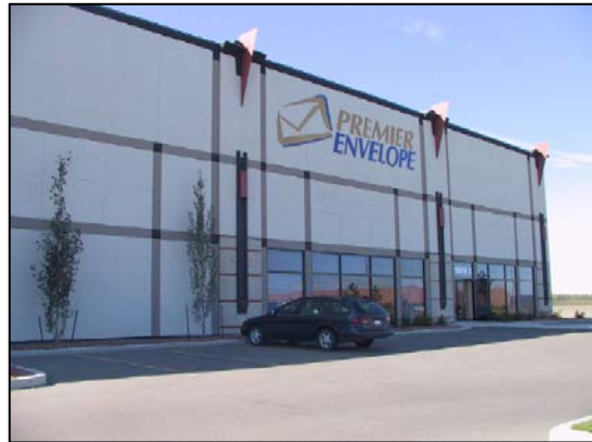
Buildings are encouraged to use multiple colours on exterior finishes. Vertical columns and landscaping can be used to break up large, uniform wall surfaces.
